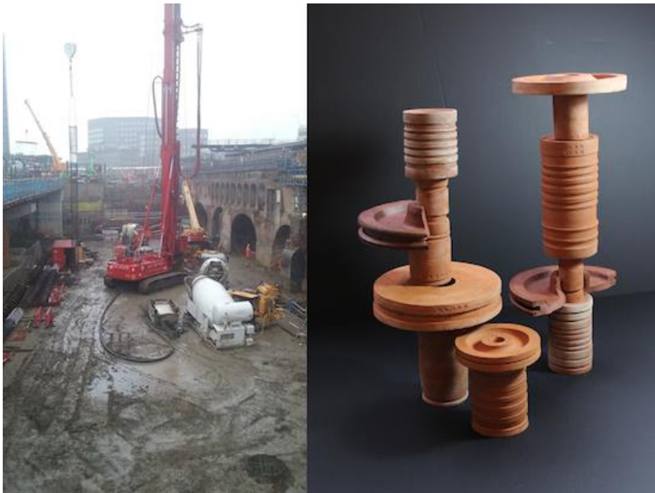
Fig.2. Construction site, Southwark Cathedral exhibition, Alison Cooke
