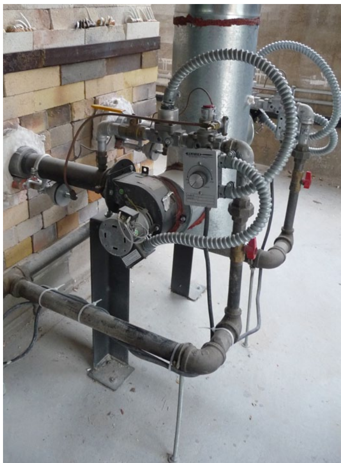
Below: Figure 10. Close up of Ward MB-200 blower burners and the preheated air duct.
